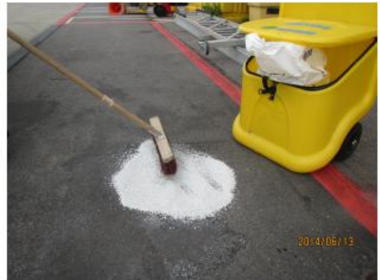
2. Work it in using a broom. Repeat the procedure until the surface is clean and dry
